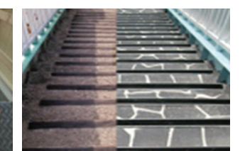
Repairing of deteriorated nonslip
